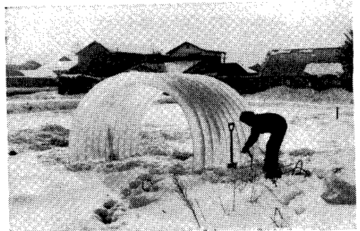
pumping up a line of tubes
