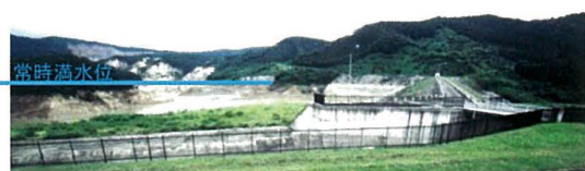
Fig. 23 貯水池越しの左岸上流地山の山体崩壊 Destructed area by landslide over reservoir of Aratozawa Dam
