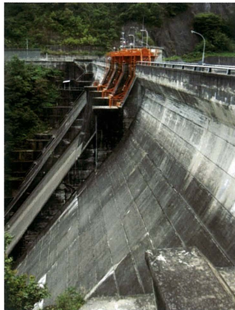
Fig. 52 豊沢ダム Overall view of Toyosawa Dam
