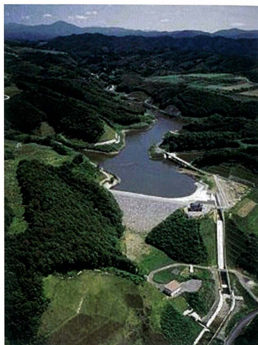
Fig. 54 相川ダム Overall view of Aikawa Dam
