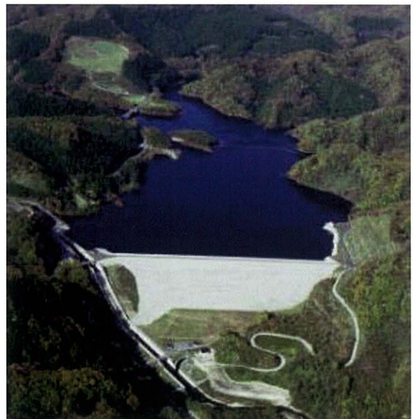
Fig. 60 ニツ石ダム Overall view of Futatsuishi Dam
