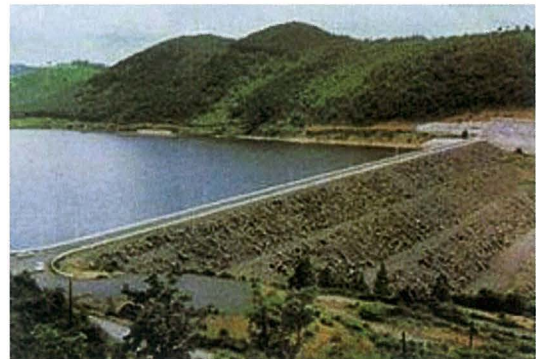
Fig. 44 岩洞ダム Overall view of Ganndou Dam
