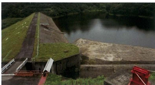
Fig. 14 川西ダム Overall view of Kawanishi Dam
