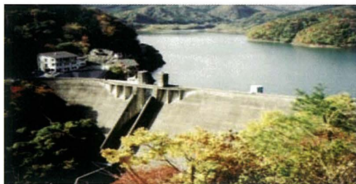
Fig. 29 栗駒ダム Overall view of Kurikoma Dam
