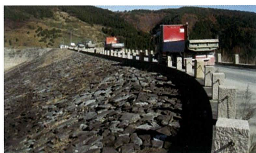
Fig. 25 流入土砂排土運搬用のダンプカー Dump truck for excavation on the crest of Aratozawa Dam
