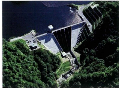
Fig. 56 岩堂沢ダム Overall view of Gandouzawa Dam
