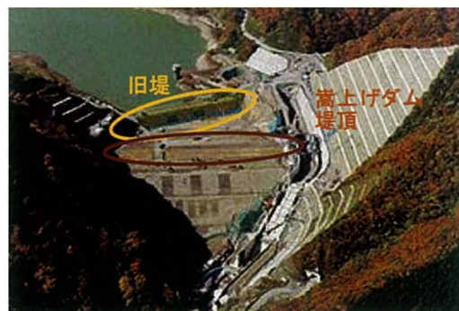
Fig. 48 旧山王海ダムと嵩上げ山王海ダム Overall view of old Sannoukai Dam and raising Sannoukai Dam
