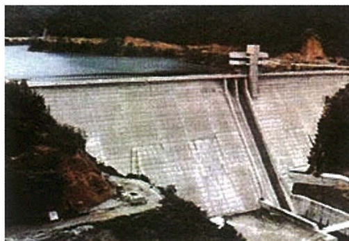
Fig. 33 柘沢ダム Overall view of Masuzawa Dam
