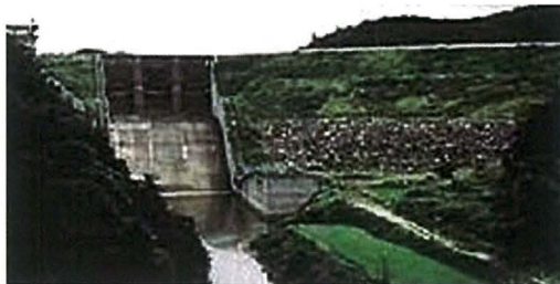
Fig. 66 千五沢ダム Overall view of Senngosawa Dam
