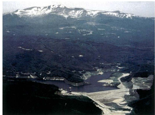
Fig. 21 荒砥沢ダム Overall view of Aratozawa Dam
