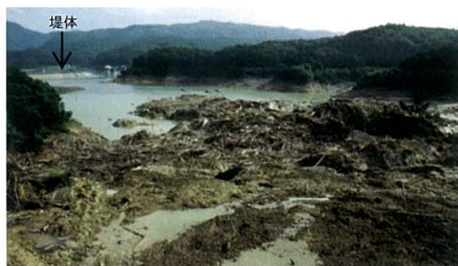
Fig. 24 貯水池に流入した崩壊土砂 Inflow of destructed area by landslide into reservoir of Aratozawa Dam
