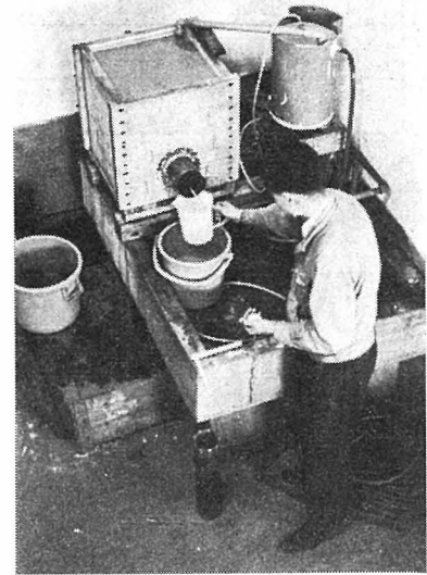
Fig. 3. 吸水率測定状況 Measurement of drainage effectiveness
